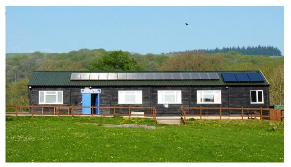
ABOVE: The Longmynd Adventure Camp Mess hall roof - to the right 3 rail mounted Vaillant Flat Plate Solar Collectors to heat water for the Kitchen and a small wheelchair friendly ablutions facility - in the centre an array of 16 Sanyo HIT250 Solar PV Modules to generate electricity. In October 2011 the Trustees reported that the system generated over 2,300 kWh of electricity in the first five months of operation worth over £1,050 in FIT payments. The Camp's electricity bills were also reduced.
