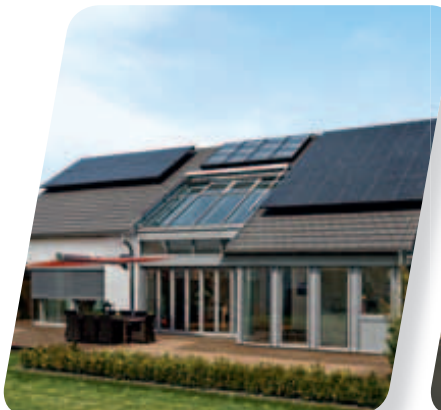
Öschelbronn, Germany: House with Suntech modules
